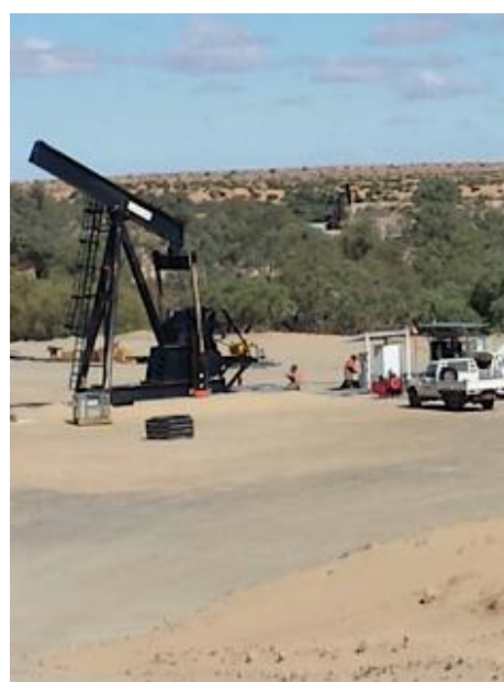
Pump installation at Spitfire
