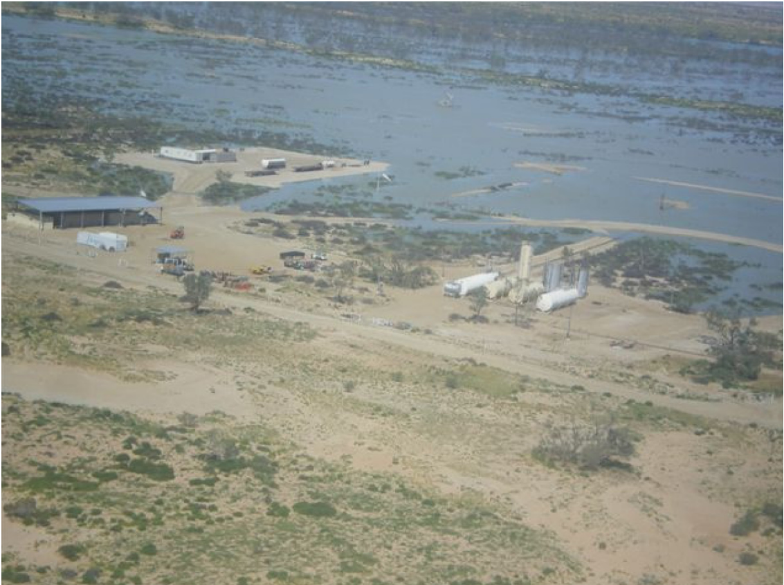
Photo 1 – Growler Oil Field Central Production Facilities, March 2010
