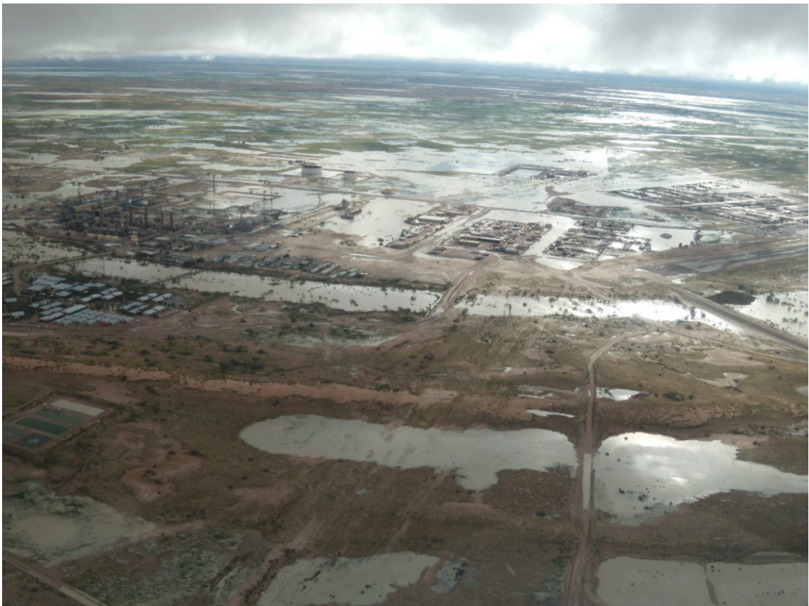
Photo 2 – Moomba Production Facilities, February 2010
